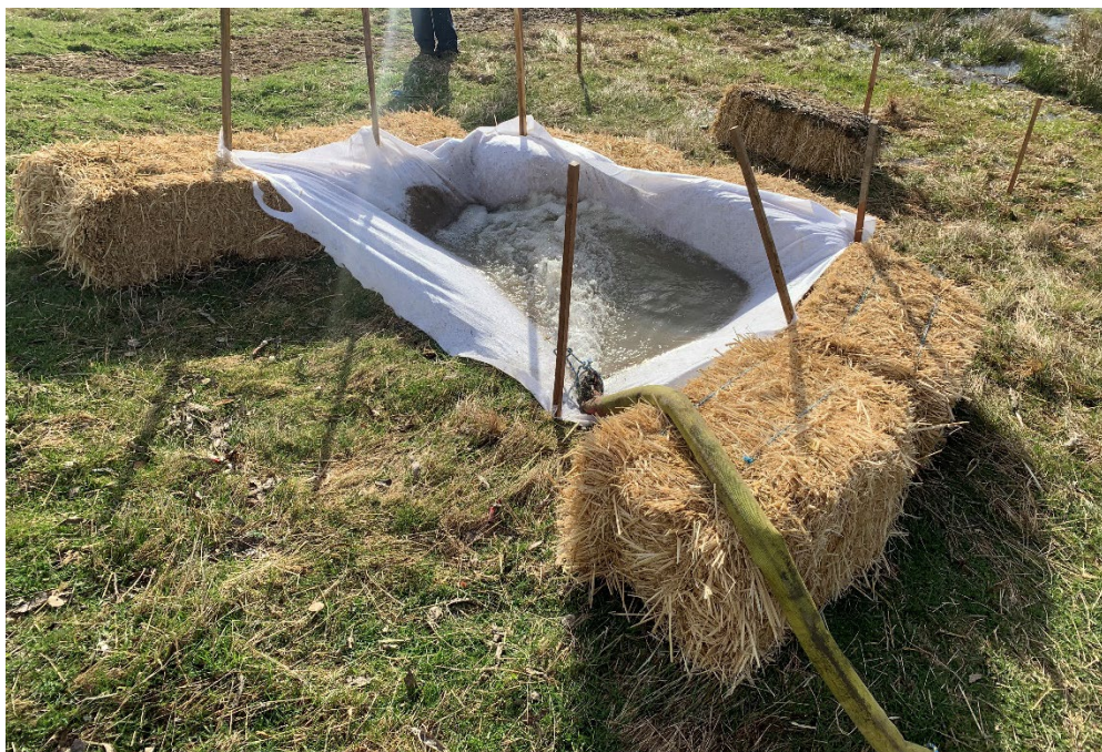
Figure 4: Standard Installation of Geofabric Filter Dam
