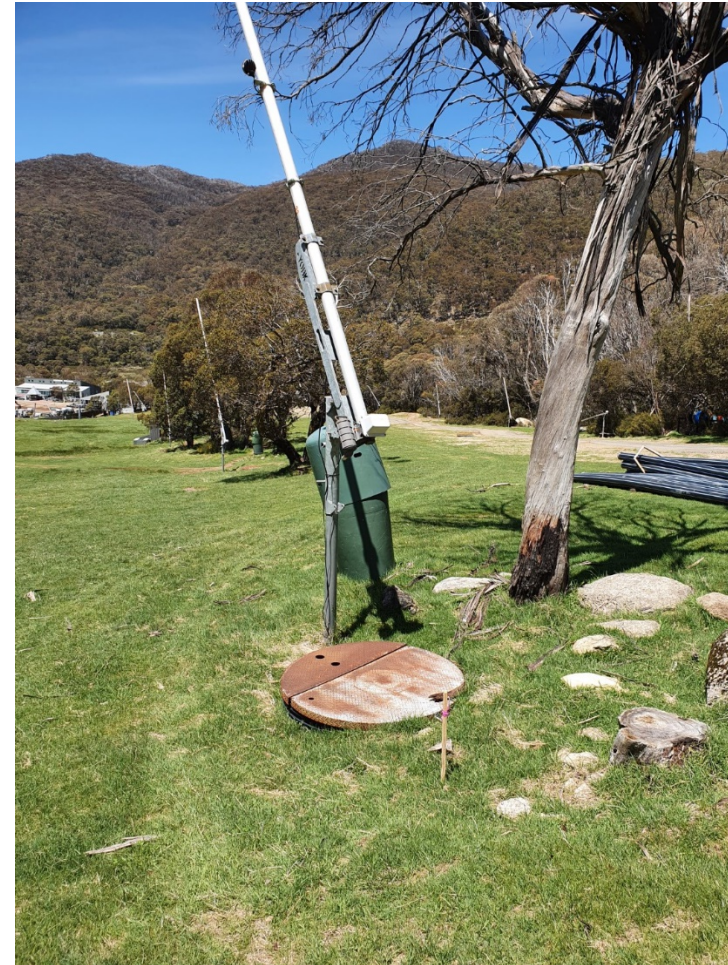
Photo A5: TT10 #3 (Easy Does It, skiers right) – replacement of existing lance gun with TT10 fan gun
